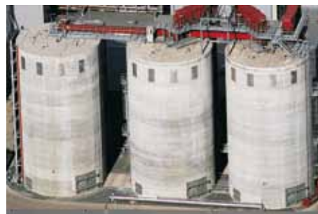
Concrete silo plant for wood chips
